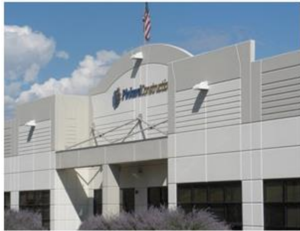
Garrison Business Park, Lakewood, Colo.
