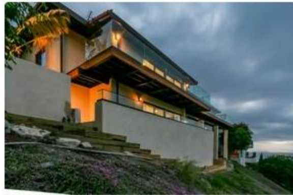
A home in Rancho Palos Verdes recently acquired and renovated by Pathfinder Partners of San Diego. -- Photo courtesy of Pathfinder Partners LLC
