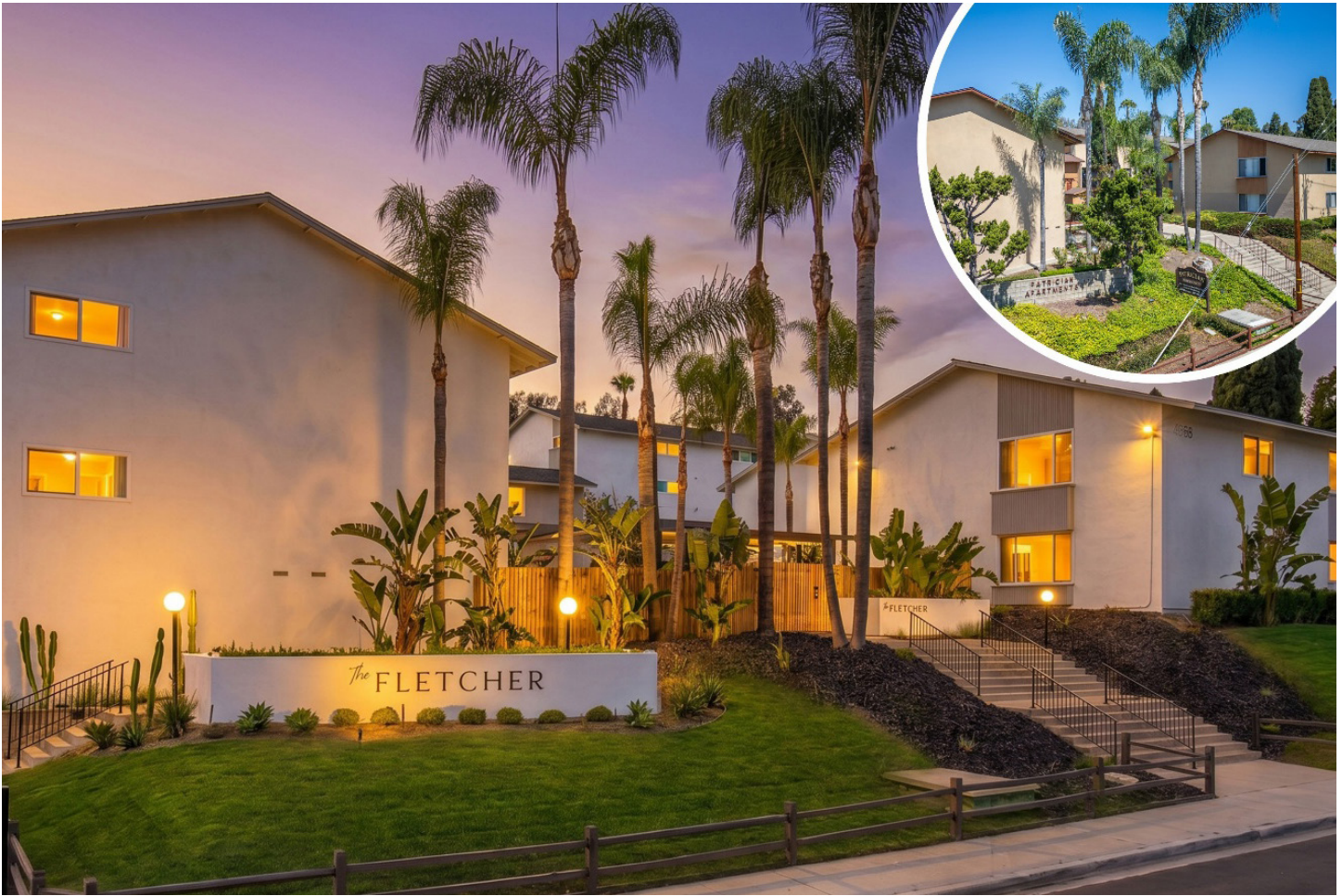
Before and After Renovations –Façade at The Fletcher
